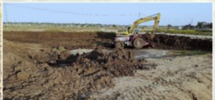
2.5m trench due to subtropical climate
