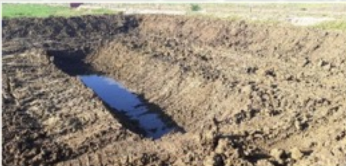
Grow-out pond under construction
